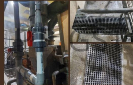
REPLACEMENT VALVE PVC & INSTALL SMALL FRP GRATING BACK AREA PICKLING
