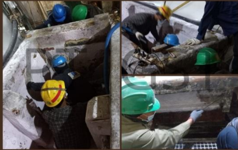
Repair Phospate Tank FRP
