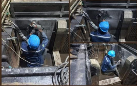
Repair Avid Tank 1 Area Pickling Material FRP
