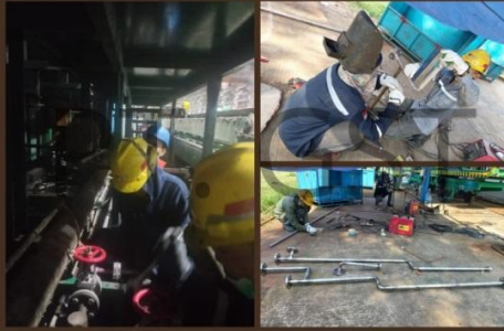
REPLACEMENT STEAM PIPE BNS OIL
