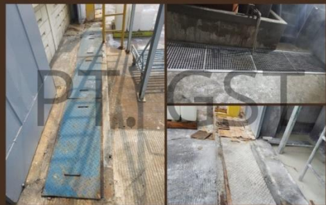
Replacement Walk Way Front Boilerroom and Extension For Chemical Loading
