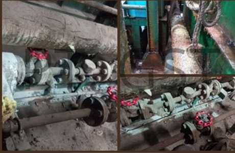
REPLACEMENT STEAM PIPE BNS OIL
