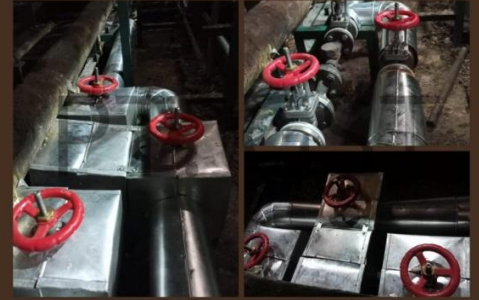
REPLACEMENT STEAM PIPE BNS OIL
