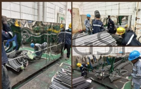
Cover Blower Boiler Room Draw Bench
