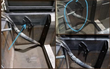
Repair Avid Tank 1 Area Pickling Material FRP
